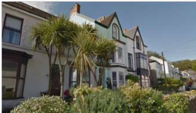
The range of Victorian and Edwardian designs of properties introduces variety and interest along the edge of the Conservation Area
