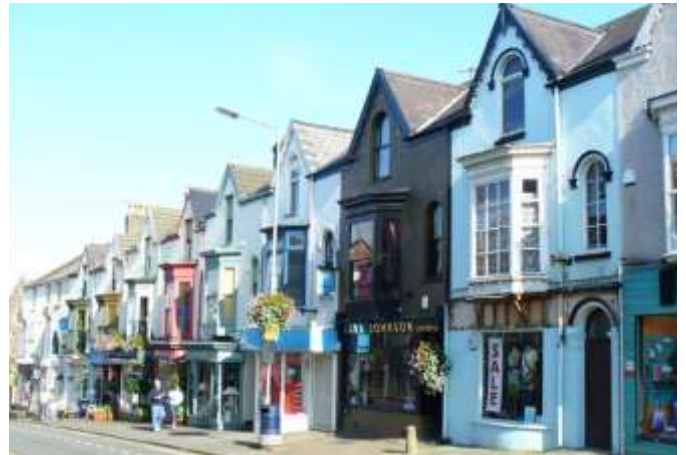
An example of the typical terrace of shops in this Character Area. The gable dormers and first floor bays create the attractive characteristics of this streetscape and limit the impact of the loss of heritage details on many buildings – chimney pots and stacks, decorated bargeboards, replacement fenestration with variety of designs, and inappropriate shopfronts and doors.
