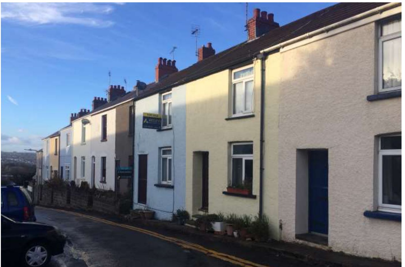
Top of Thistleboon Road showing the traditional two storey terraces stepping down the hill. Narrow roadway and problems for parking throughout the Character Area.
