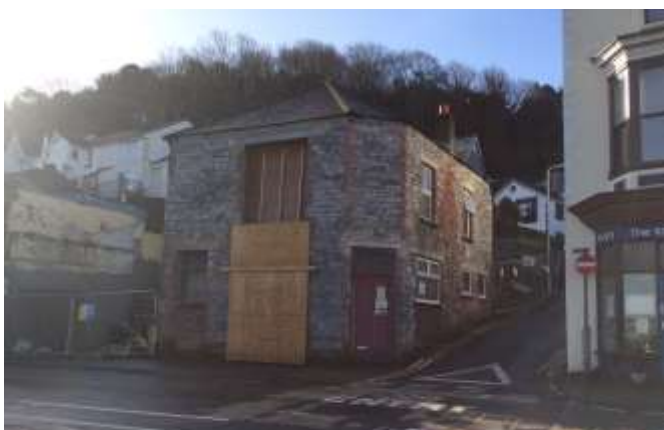
Longstanding vacant buildings can detract from the visual qualities of the heritage environment
